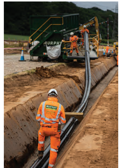
Image 3 shows trenching and cables being laid
