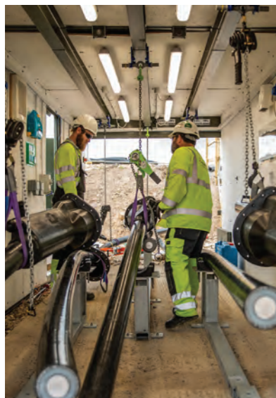
Image 1 shows two lengths of cable being safely jointed
