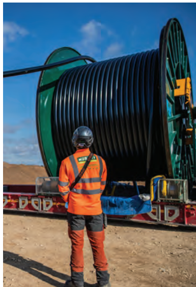
Image 2 shows delivery of a reel of cabling
