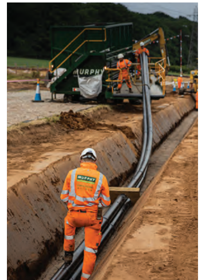
Image 3 shows trenching and cables being laid
