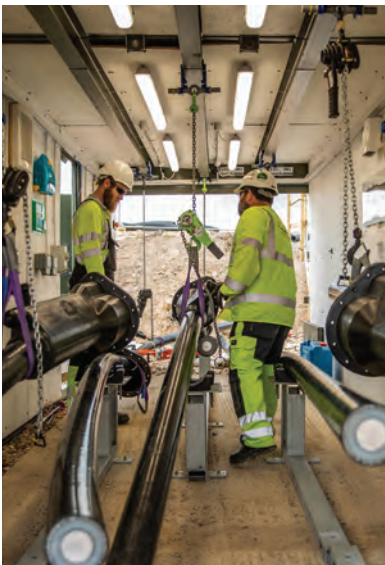
Image 1 shows two lengths of cable being safely jointed
