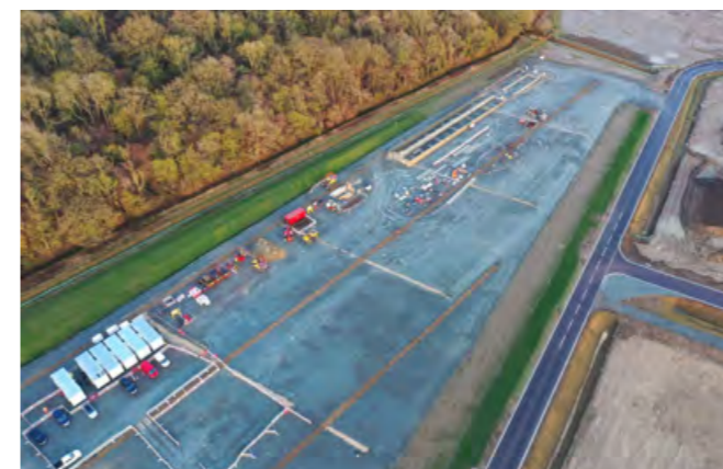
New contractor compound
