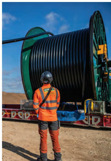
Image 2 shows delivery of a reel of cabling
