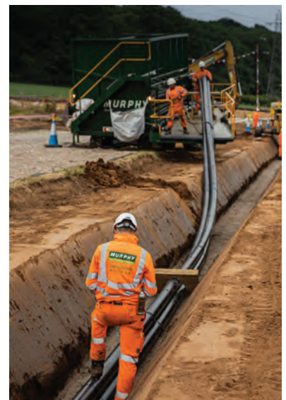
Image 3 shows trenching and cables being laid
