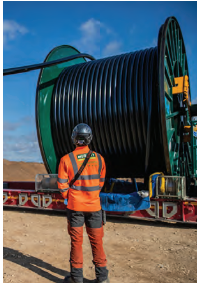
Image 2 shows delivery of a reel of cabling
