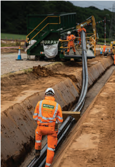
Image 3 shows trenching and cables being laid
