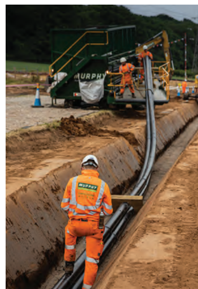
Image 3 shows trenching and cables being laid
