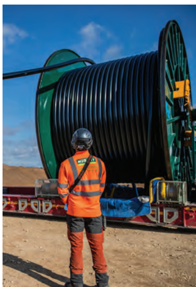
Image 2 shows delivery of a reel of cabling
