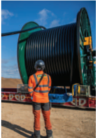
Image 2 shows delivery of a reel of cabling
