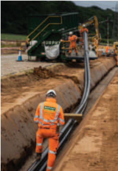
Image 3 shows trenching and cables being laid
