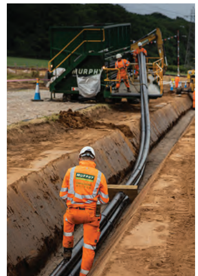
Image 3 shows trenching and cables being laid
