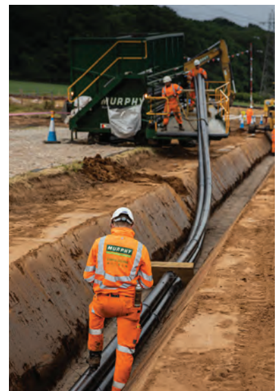
Image 3 shows trenching and cables being laid
