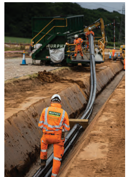
Image 3 shows trenching and cables being laid
