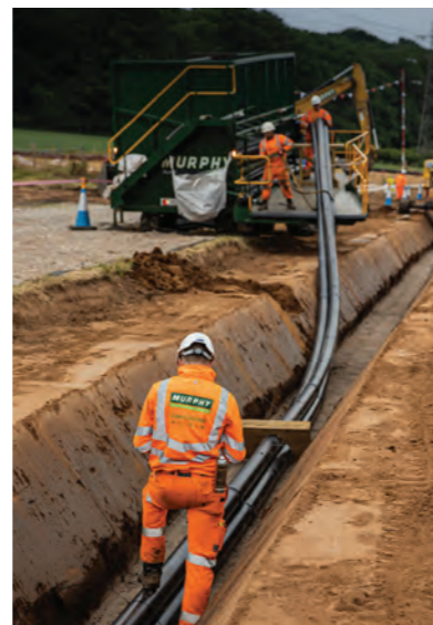
Image 3 shows trenching and cables being laid
