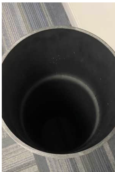
The ducting has a diameter of 225mm
