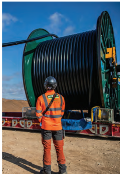
Image 2 shows delivery of a reel of cabling
