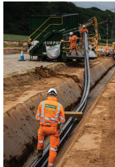
Image 3 shows trenching and cables being laid
