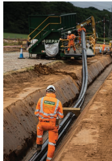
Image 3 shows trenching and cables being laid
