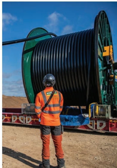
Image 2 shows delivery of a reel of cabling
