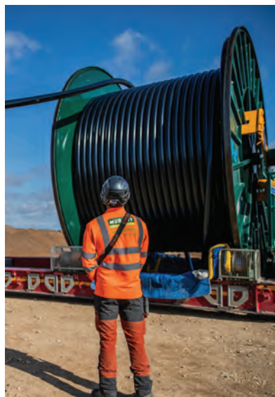
Image 2 shows delivery of a reel of cabling
