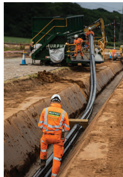
Image 3 shows trenching and cables being laid
