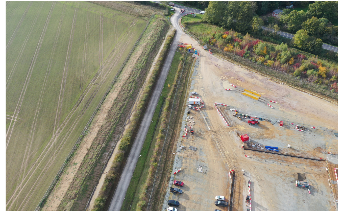
AC178 access road
