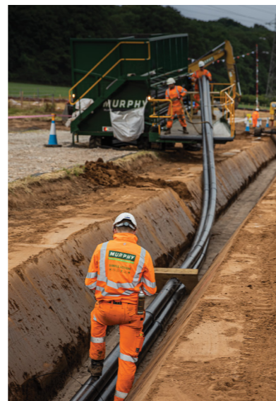
Image 3 shows trenching and cables being laid
