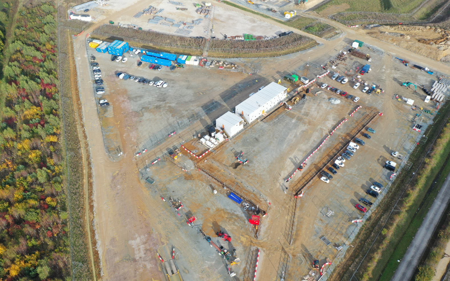
400kV site establishment
