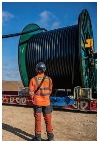
Image 2 shows delivery of a reel of cabling
