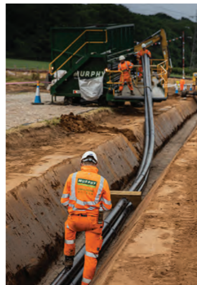
Image 3 shows trenching and cables being laid
