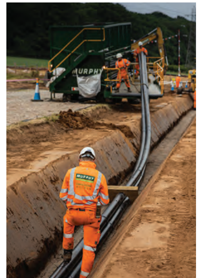
Image 3 shows trenching and cables being laid
