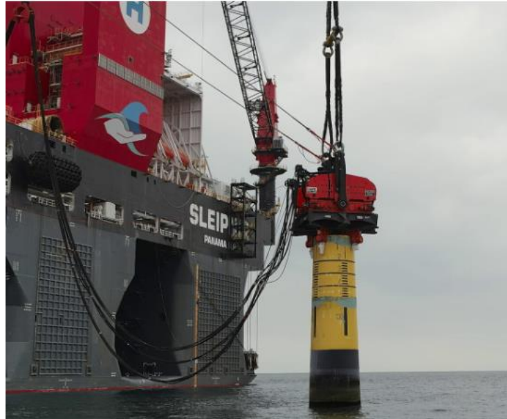
Figure 6-1: Vibro extraction carried out by CAPE HOLLAND 9
