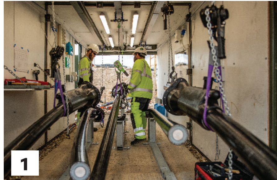
IMAGE 1 SHOWS TWO LENGTHS OF CABLE BEING SAFELY JOINTED
